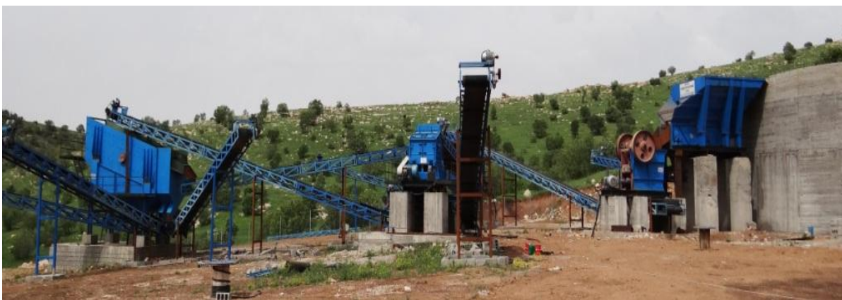
Figure-3: Tlazait Crusher.
